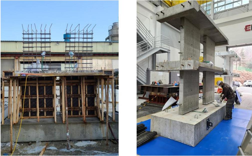
**Fig. 1** Construction of Specimen
